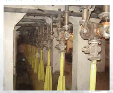
The heating fittings are intended for coke or blast furnace gas supply from the collector to the heating system of coke ovens as well as air supply for degraphitization of gas supplying As per the method of heating gas supply, the fittings are split up into heating fittings for the ovens with the lower system of coke gas supply and with the side system.
